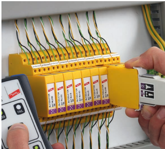
Figure 12 Combined arrester modules with LifeCheck
