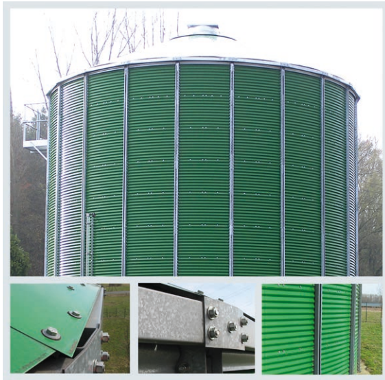
Figure 6 Fermenter made of bolted metal sheets
