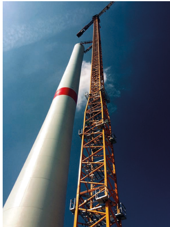
Figure 1 Hybrid tower made of pre-fabricated concrete elements
