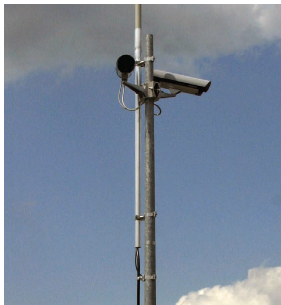
Figure 4 HVI Conductor installed at a pylon
