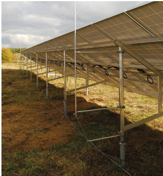
Figure 2 Lightning protection by means of DEHNiso spacers
