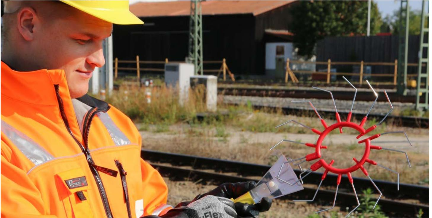
With the new adapter AD ZK 3M 170 the Animal Guard™ 3M bird and small animal deterrent can be mounted quickly and easily on insulators. You prevent arcs that lead to the death of birds and small animals by electric current. Railway traffic is not disrupted by earth faults and short-circuits.
