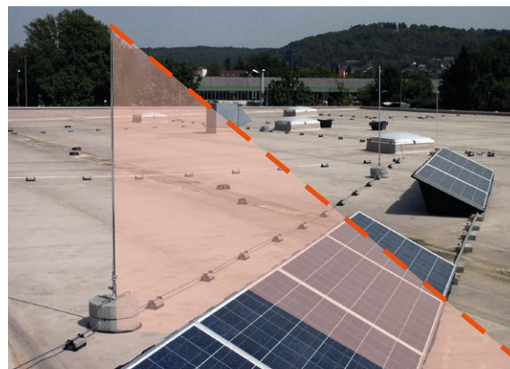
Figure 12 Determination of the protected volume using the protective angle method
