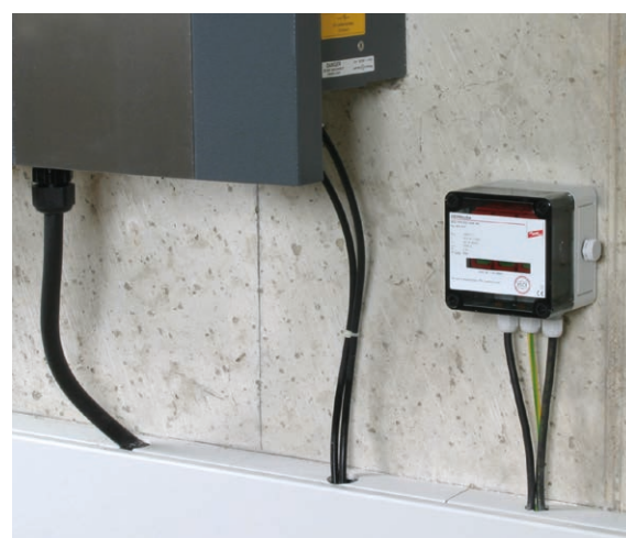
Figure 14 DEHNcube YPV SCI 1000 1M type 2 arrester for protecting inverters (1 MPPT)
