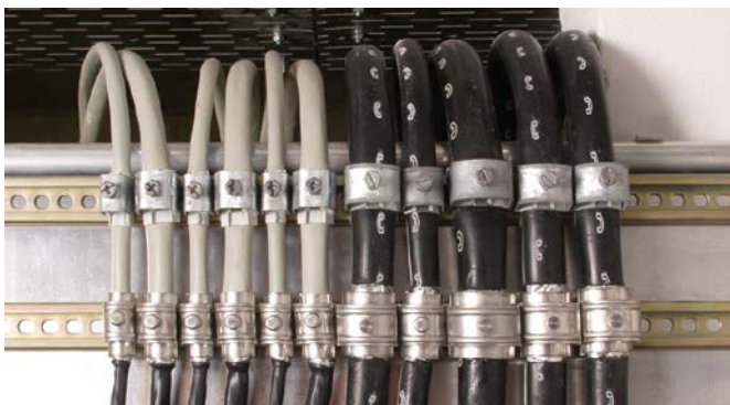
Lightning current carrying shield connection system for anchor bars. A slipping spring element compensates the yield of the cable materials used.
