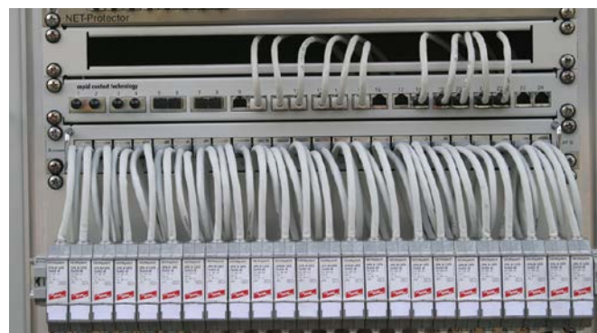
DEHNpatch is the first Cat. 6A certified patch cable with surge protection that can be used according to IEEE 802.3at up to 57 V.
