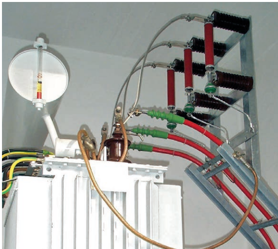
Figure 10 DEHNmid: surge arrester for medium-voltage systems
