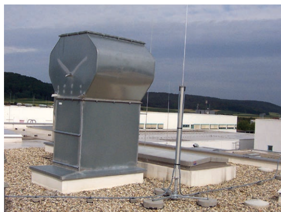
Figure 3 Isolated lightning protection with HVI-light conductor
