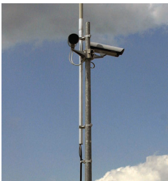
Figure 4 HVI Conductor installed at a mast
