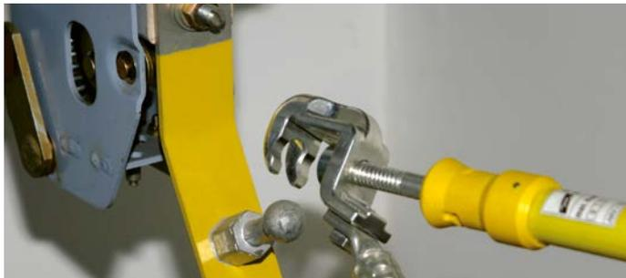
Installation of an earthing and short-circuiting device with universal clamp for fixed ball points (20 or 25 mm)
