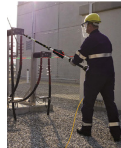
Testing with HS 36 in a 36 kV distribution panel
