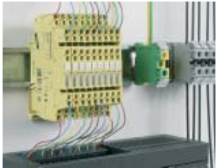
Protection of PLC* in-/outputs*
