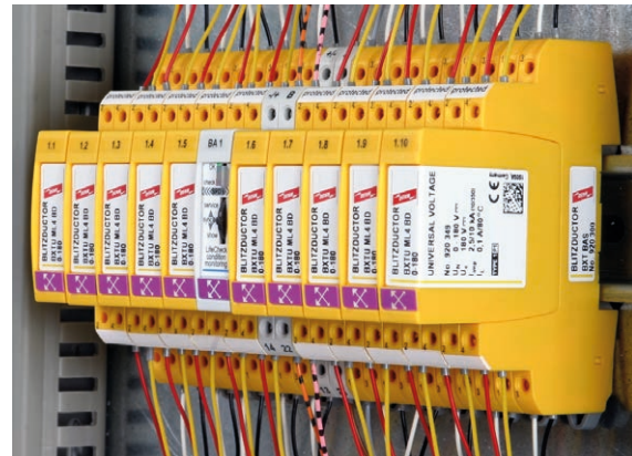
Figure 12 BLITZDUCTOR: combined arrester with actiVsense technology and integrated LifeCheck monitoring
