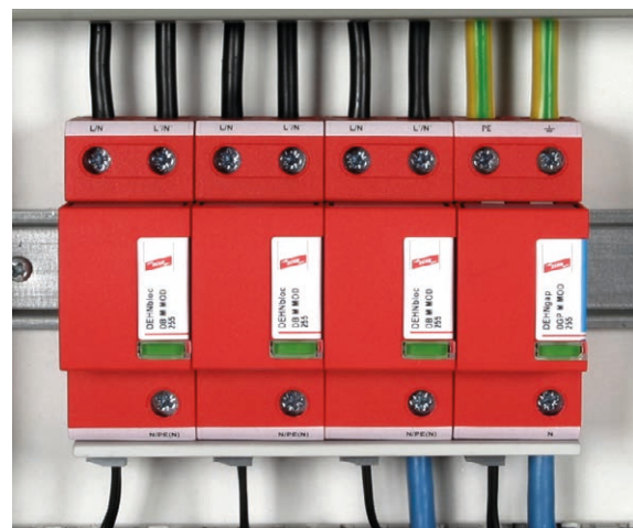
Figure 6 DEHNbloc modular: coordinated spark-gap-based lightning current arrester
