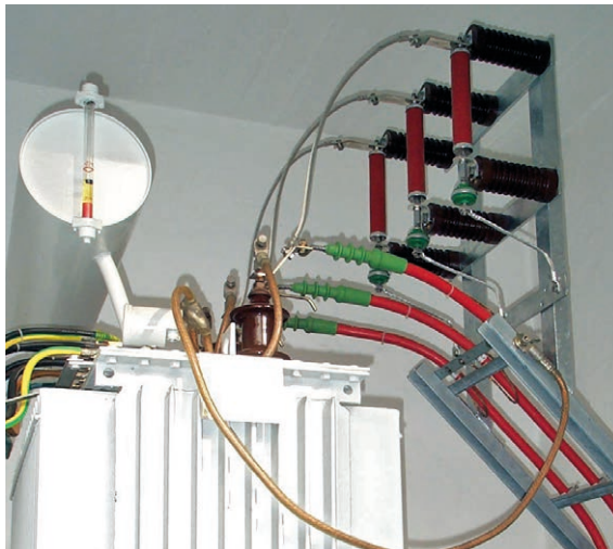
Figure 10 DEHNmid: surge arrester for medium-voltage systems
