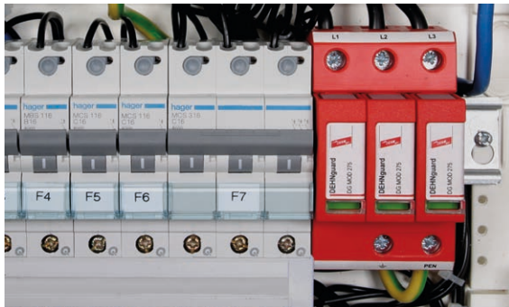
Figure 6 Modular type 2 surge arrester for protecting the 230/400 V supply
