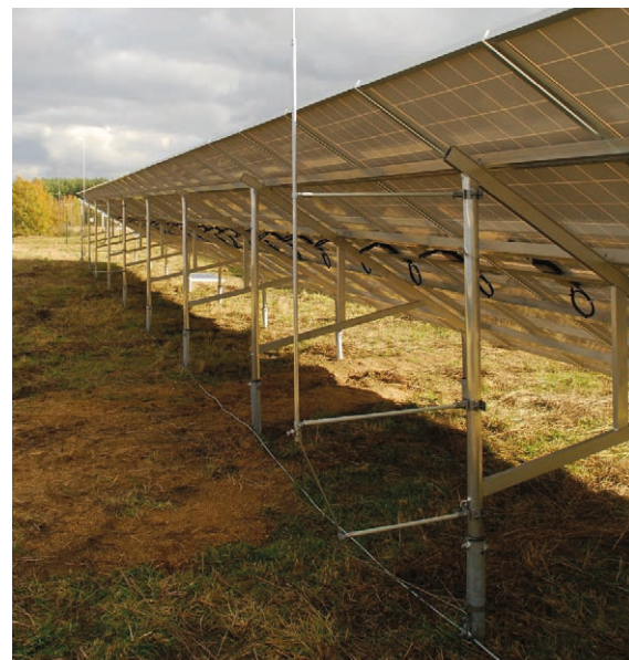
Figure 2 Lightning protection by means of DEHNiso spacers
