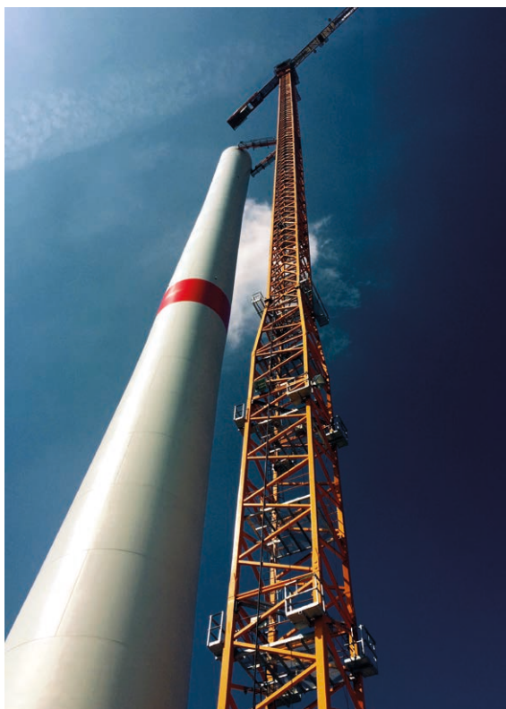
Figure 1 Hybrid tower made of prefabricated concrete elements
